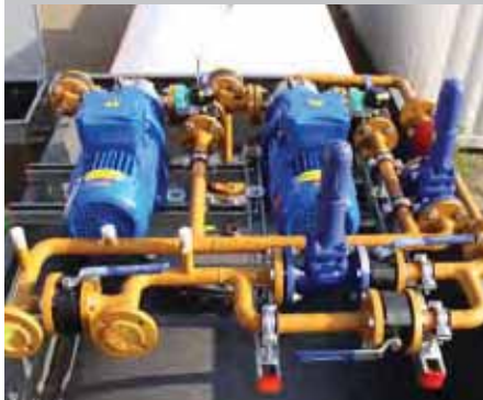
Doppelpumpenstation Pentantank double pump station pentane tank
